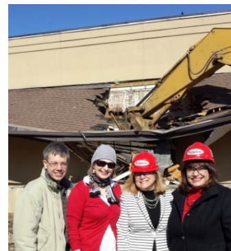
Frasier Paper plant demolition, West Carrollton
